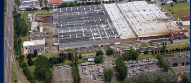
Metz: gearboxes plant
